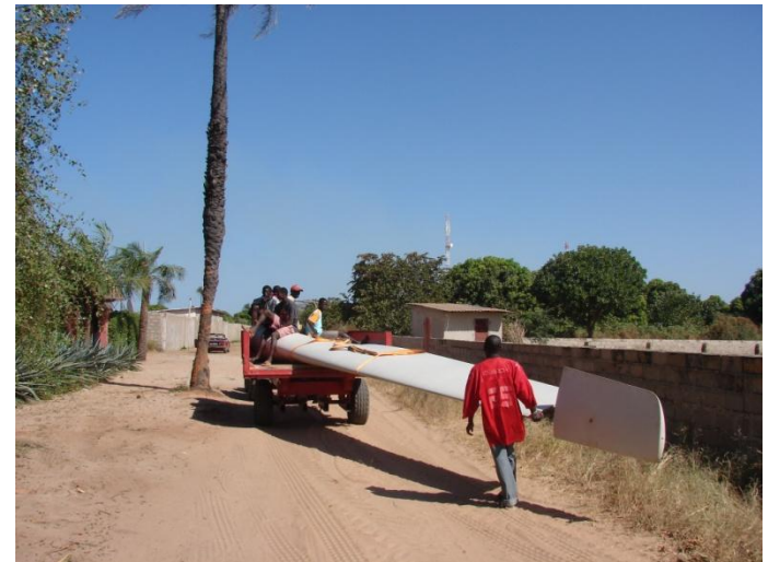
Construction of a Wind Farm in The Gambia
